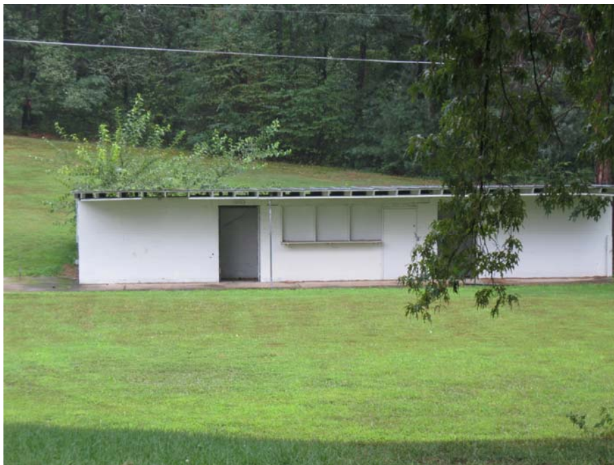
Former Outdoor Bathhouse – American Legion
